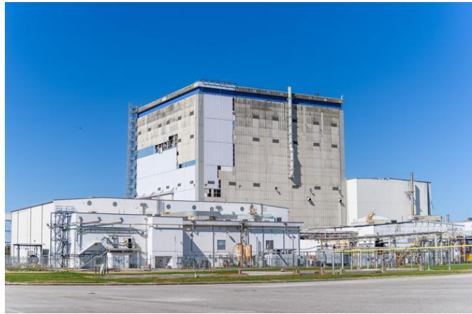
(NASA Photo) Storm Damage at Michoud Assembly Facility
