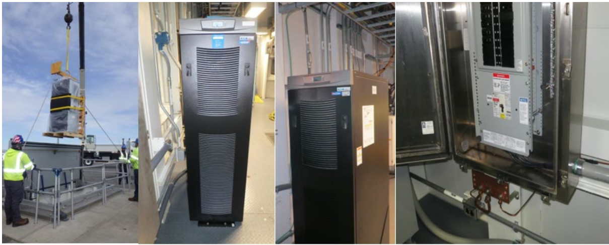
Figure 2: SIV UPS Hardware Installation and Checkout
